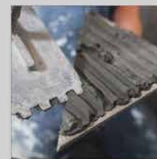
Cement Laying On Tile
