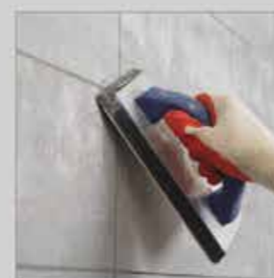
Joint Grouting
