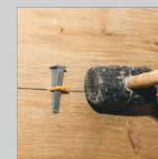
Remove Wedges Ones If Dry
